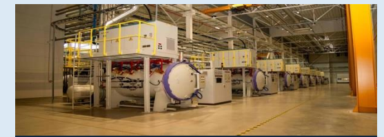
Neo's NdFeB magnet plant, Narva (EE) — operating since 2025
